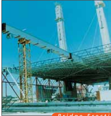
Bridge Erection & Tensioning
